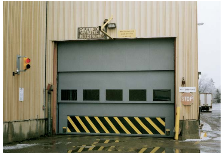
Vertical Lift with Break Away Panel
